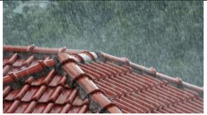
Rain falling on a roof
